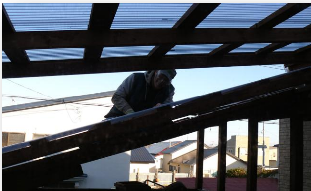
Adding adjustabel 'roofing' to the deck for snow removal
